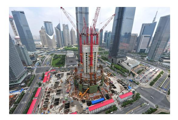
in the engineering management of this project, reflecting a new mode of digitalized management. Digital construction technologies were widely applied to construction site planning, including pile positioning using the reverse construction method; studies related to environmental impact of confined water, environmental impact of foundation pit construction and visualized monitoring; crack monitoring of mass concrete; steel structure processing and use of the welding robot; mechanical and
